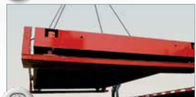
2 Unload and set modules.
