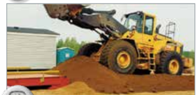
3 Backfill to bulkheads and finish ramps.
